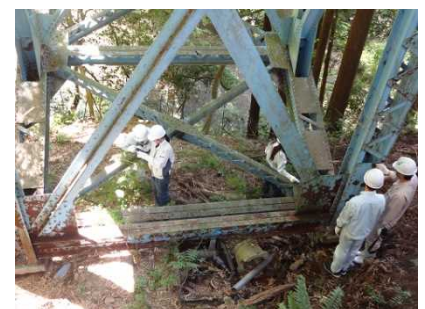
Field investigation of an aging bridge
